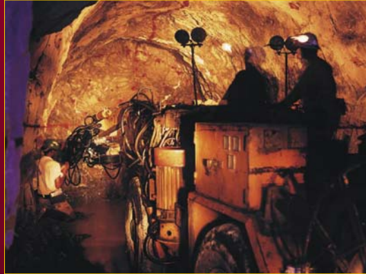
Jumbo drill rig
